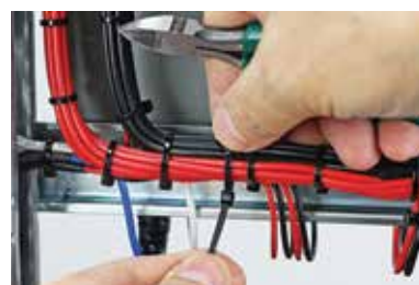
Figure 3: Selecting correct size cable tie supports airflow within enclosures, helping to reduce localised heat accumulation.
