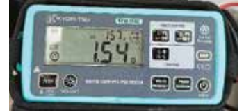
(d) Earth loop impedance test -- Earthing rods with connection to foundation steel re-inforcing bars
