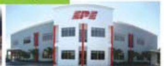
EPE Switchgear, Nilai Sizes: 176 kWp
