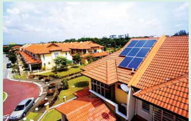
Solar Photovoltaic (PV) rooftop setups for businesses and homes.
