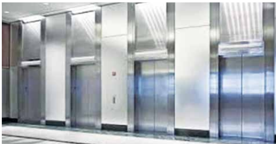
Figure 1: A typical lift arrangement in a modern building complex.
