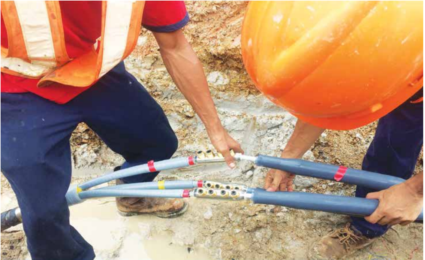
HV Cable Jointing.
