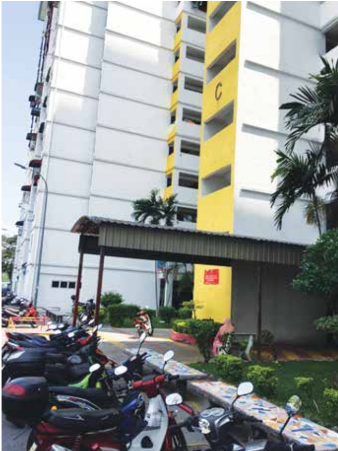
Figure 2: The Block C, PPR Kerinchi Pantai Permai flats where the lift accident was reported.
