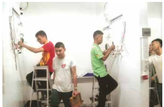
Hands-On – Trainees learning the proper wiring installations.
