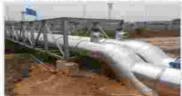
KLIA2 - 4700m underground infra distribution 1000mm diameter Chilled Water Pipework
