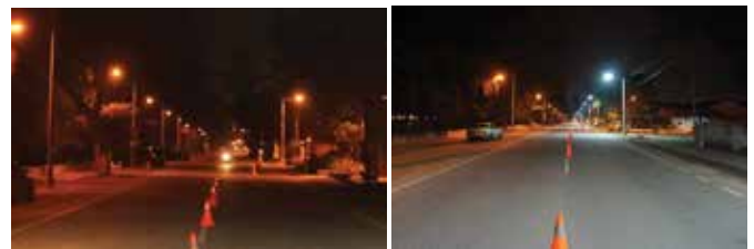
Figure 2: Induction Street Light before and after installation
