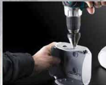
Box walls without knock outs can be individually drilled for cable entries
