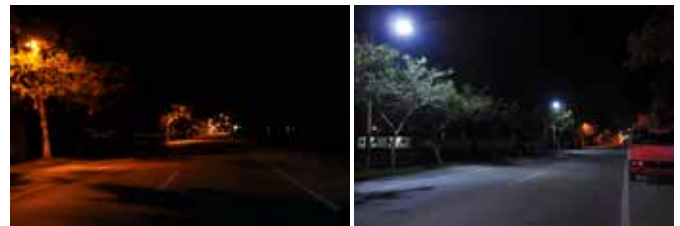
Figure 1: LED Street Light before and after installation
