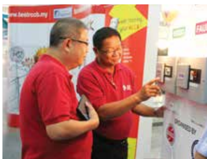
Safety awareness – Mr Francis Chew of SEA demonstrates on how to self-test RCCB.
