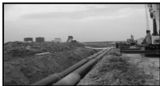
KLIA2 - 4700m underground infra distribution 1000mm diameter Chilled Water Pipework
