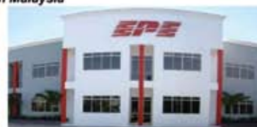
EPE Switchgear, Nilai (176 kWp)
