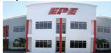
EPE Switchgear, Nilai (176 kWp)
