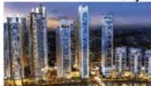
KL ECO City, Mid Valley City (40 kWp)
