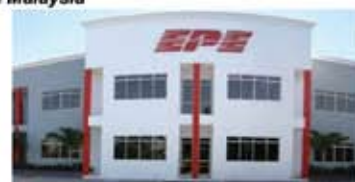
EPE Switchgear, Nilai (176 kWp)
