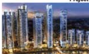
KL ECO City, Mid Valley City (40 kWp)
