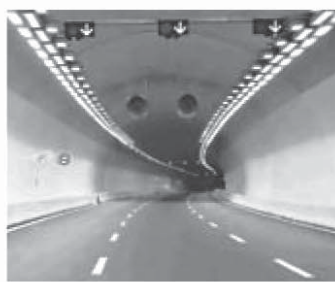
Tunnel Lighting Penchala Tunnel
