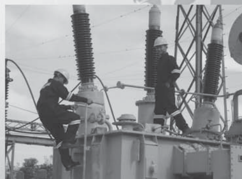
Servicing Transformer
