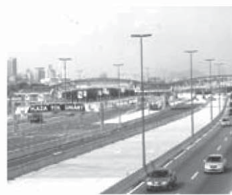
Public Lighting Jalan Sungai Besi
