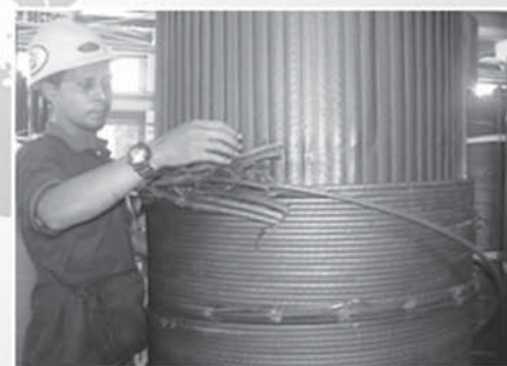
Refurbishment of Transformer
