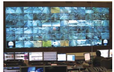
SMART Tunnel Control Room – Delegates had the opportunity to view how the SMART personnel monitor traffic flow at the tunnel.
