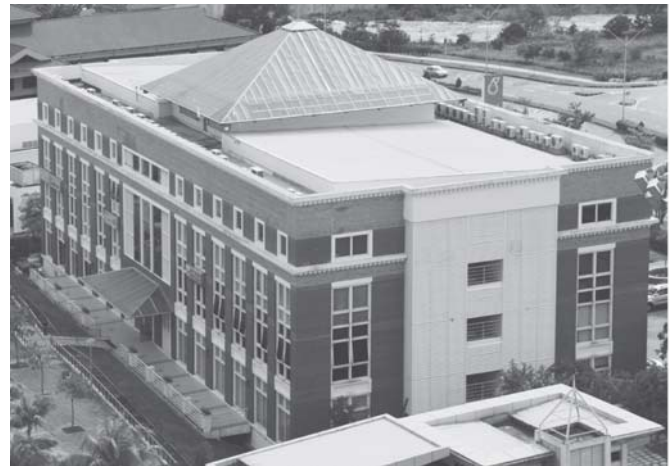
Commercial rooftop application of BIPV, Putrajaya.
