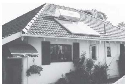
The use of solar thermal system to heat water is common in Malaysia.
