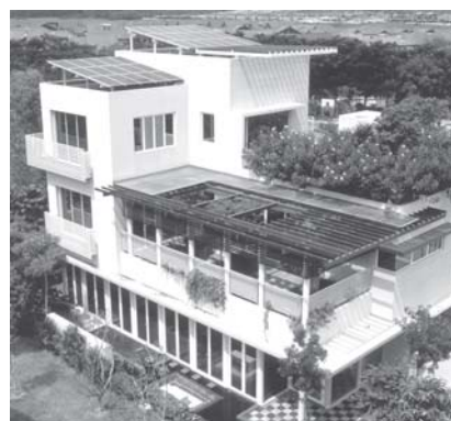
Domestic application of PV retrofitted over existing roof.
