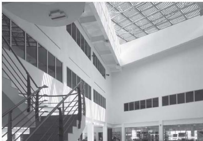
In PTM ZEO, the use of natural day lighting is maximised to reduce electricity consumption.
