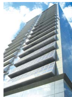
Kyocera at Kyoto - Solar power generation, one of the world's largest solar installations.
