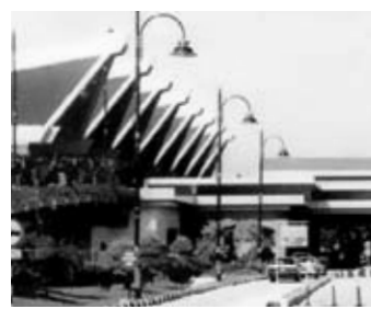
Decorative Lighting Penang International Airport
