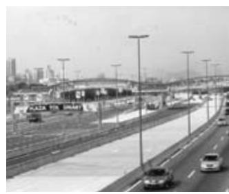
Public Lighting Jalan Sungai Besi
