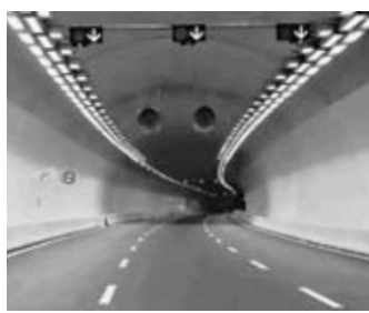
Tunnel Lighting Penchala Tunnel
