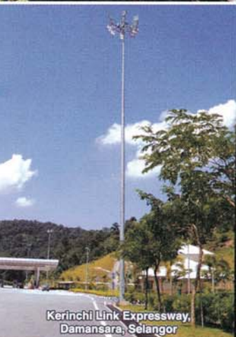
45.0m Antenna Monopole Structure
