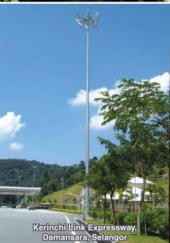
45.0m Antenna Monopole Structure
