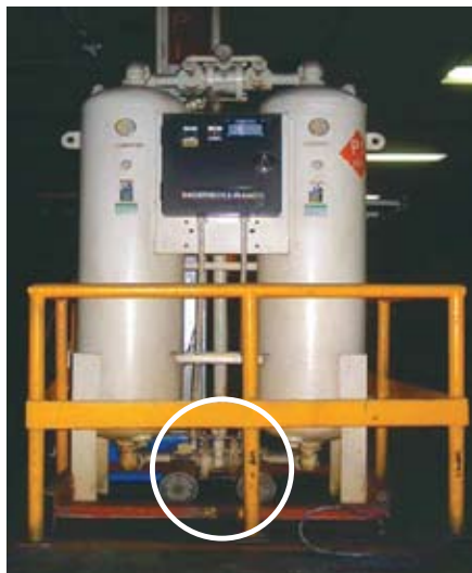
Desiccant air dryer keeps purging over night
