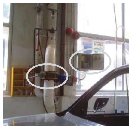
Desiccant air dryer keeps purging over night
