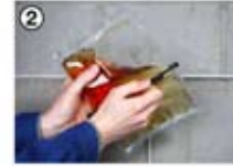
2 Remove divider between the two components of the sealing compound.
