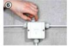
6 Insert plug, after the case has been completely sealed.
