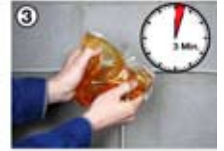
3 Mix well for three minutes the two components of the sealing compound.
