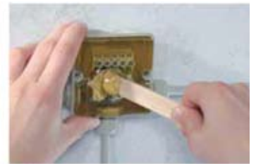
For repairs, subsequent installations or changes to installations the sealing compound can be easily removed: - Take off lid and - remove sealing compound
