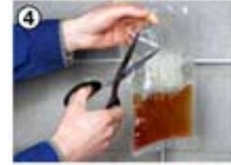
4 Cut open sealing compound bag.
