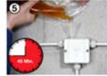
5 Use funnel for feeding sealing compound. The compound takes 45 minutes to process.
